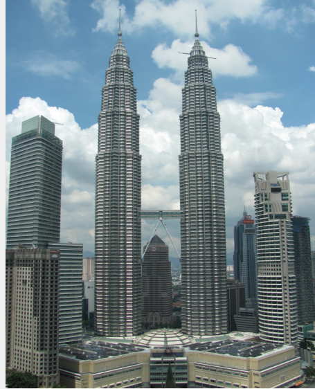
Kuala Lumpur - Twin Towers
